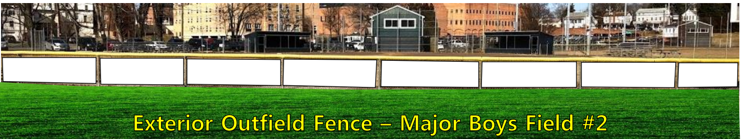
Exterior Outfield Fence – Major Boys Field #2
