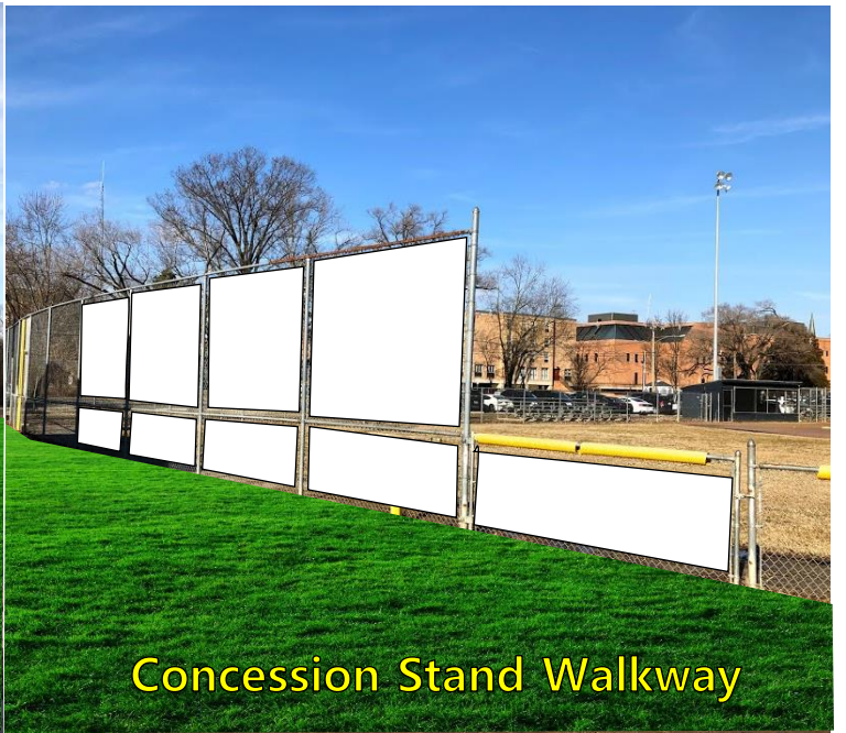
Concession Stand Walkway
